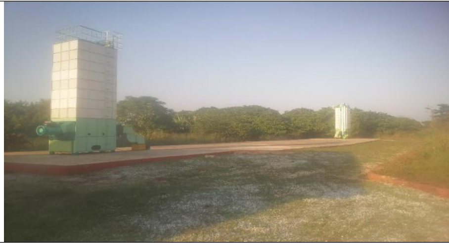
Two gas powered Dryers on a concrete platform
